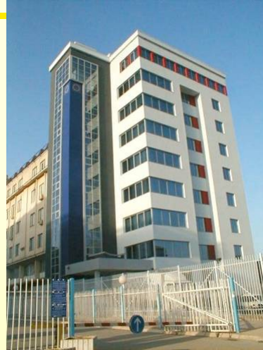
EAR Tower Pristina Kosovo 226 m 2 /160 kW/ Solar Air conditioning
